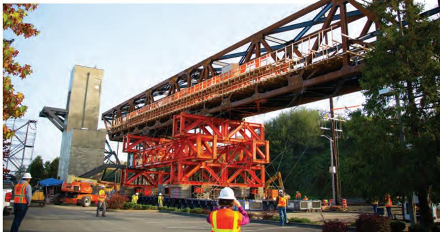
towers where it would be lifted to a height of 36 feet, building a cribbing system on a reformatted SPMT system underneath the bridge, lashing the bridge back to the cribbing and SPMT system and then moving and rotating the bridge again to be installed on its foundation on either side of the roadway.
